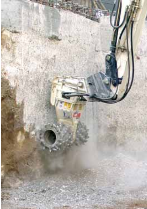
Demolitions and rough wall profiling, even with bracing, without damage to adjoining buildings.
